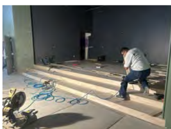
Wood Flooring at Stage
