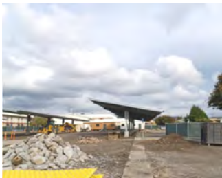
Parking Lot Demolition of asphalt
