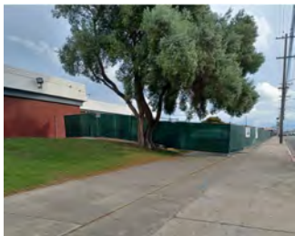
Construction Fencing Along 23rd Street
